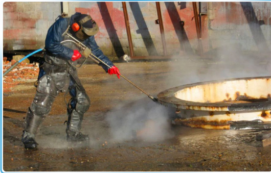
UHP Water Blasting
