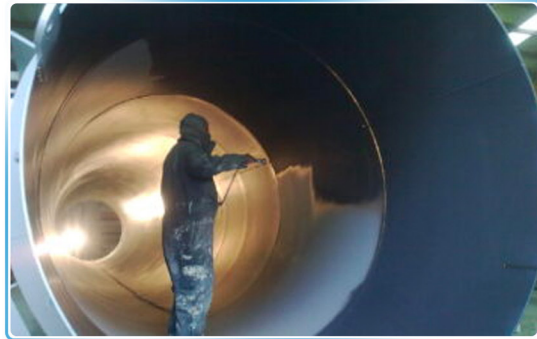
Spray painting, Industrial painting
